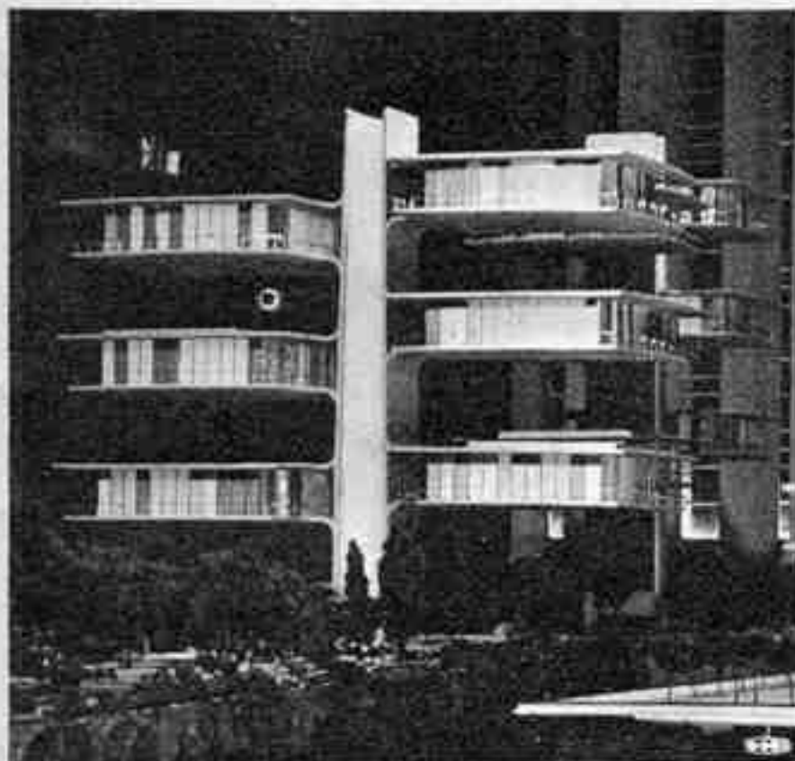
G.M.'s Futurama Building
